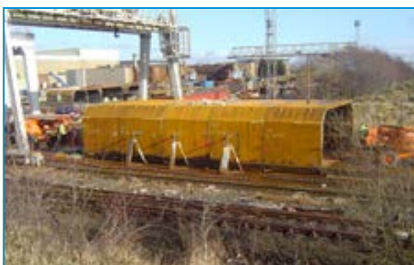
Figure A2.6 – Steel track protection structure being tested
