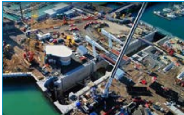
Figure A2.5 – Dock navigational access under construction
